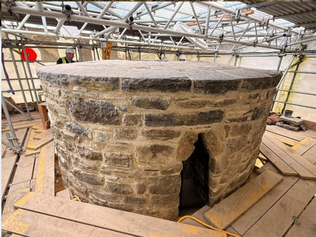
Before and After Photographs of the Round tower and cut stone capping
